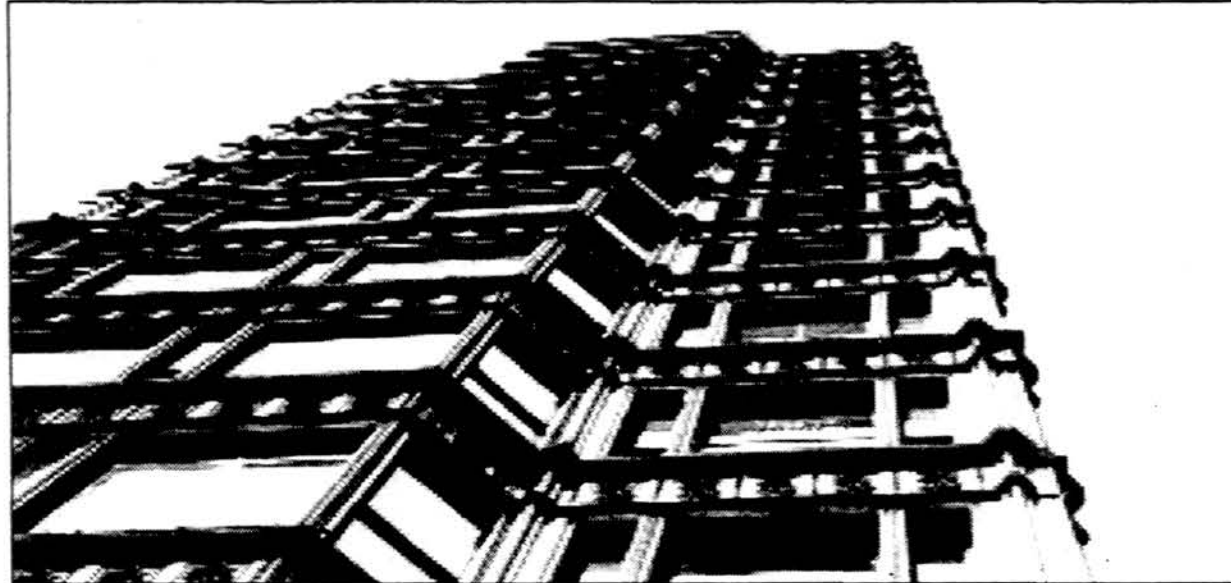
Burnham's Reliance Building, 1950 m.
